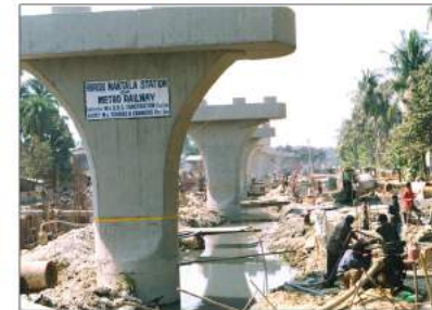
SUB STRUCTURE WORK - KOLKATA METRO
