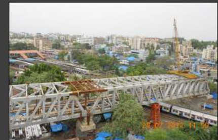
MUMBAI METRO BRIDGE - RAILWAY TRACK AT ANDHERI, MUMBAI
